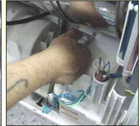
Pull out motor clamp
