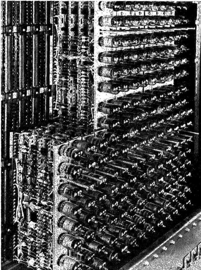
Fig. 2—Decalced tubes in 701 machine.
