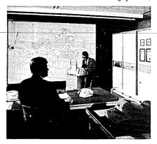
The control panel in the warning center at Schiedam shows the positions of all the measuring points in the Rijnmond region by lights.
