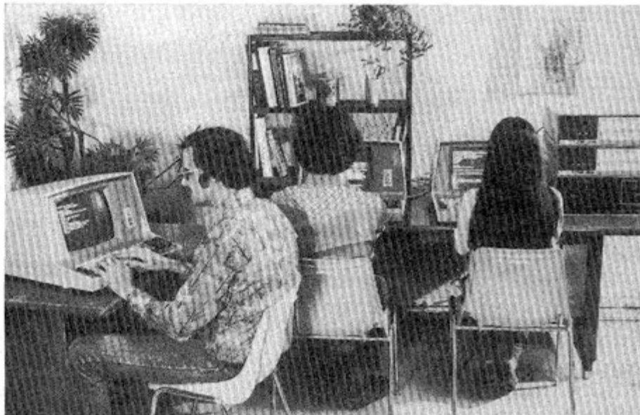
Typical Altair Timesharing BASIC system, including Altair B-100 CRTs, Altair Floppy Disks and Altair 8800b Turnkey model. Altair Timesharing BASIC supports up to eight users.
