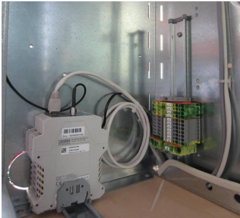
Fig. 74: UMTS router installation
