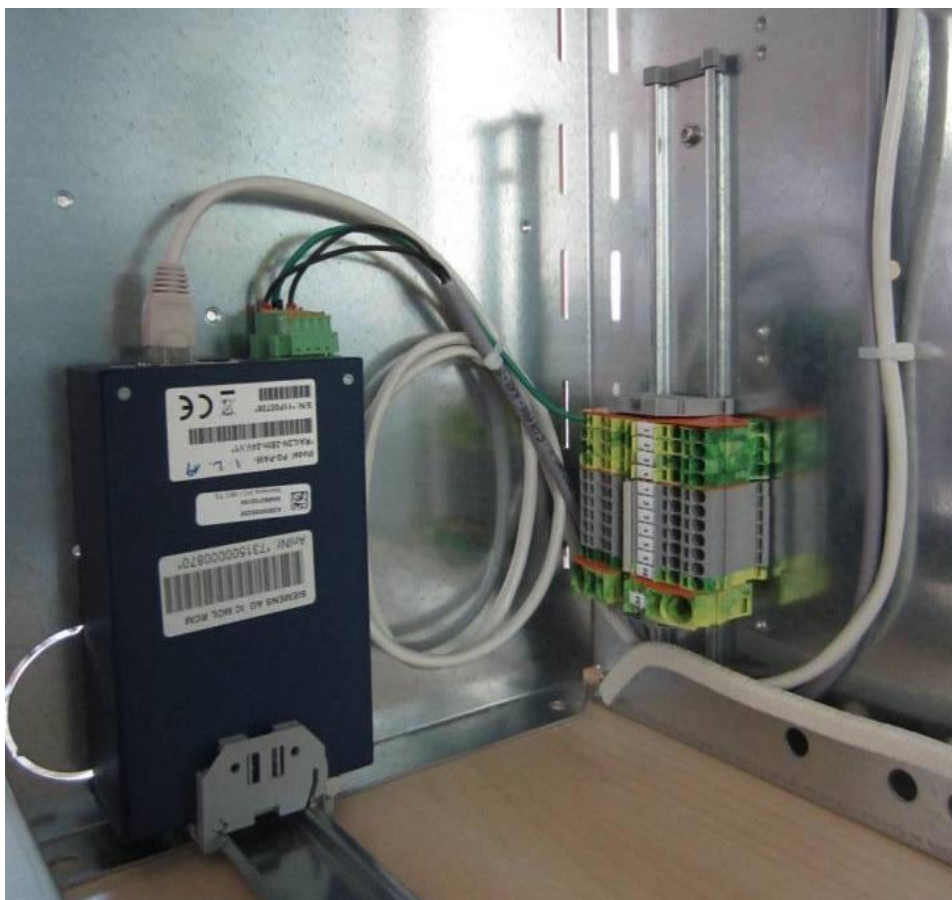
Fig. 77: Installation of Mini-Flex modem
