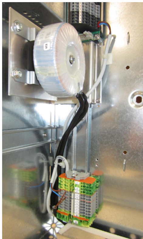
Fig. 70: Installation of the AC power supply
