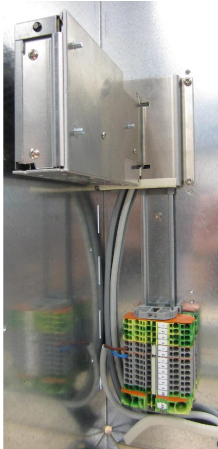
Fig. 68: Installation of the DC power supply
