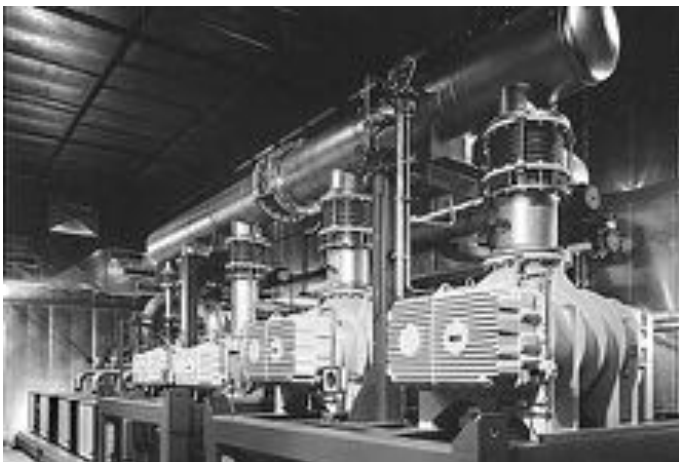
Pump system with RA Roots vacuum pumps
