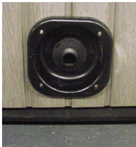
Figure 14. Cabinet mounted drain valve
