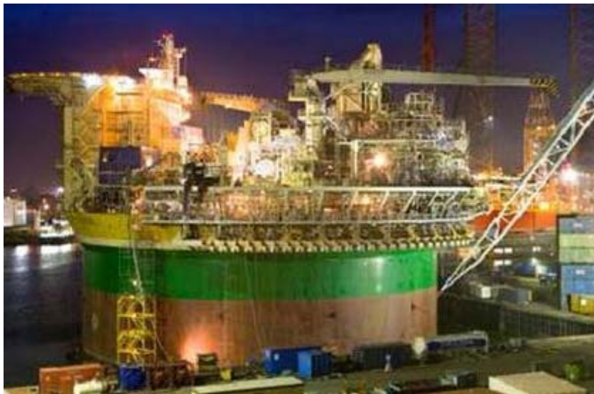
Hull No:1 at topside integration yard November 2006
