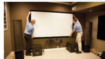
Hudson Valley Home Media techs Bart Cennamo (left) and John Mulgrew slide the Elite screen onto mounting brackets above the wall-mounted Martin Logan Cinema-i center speaker.
