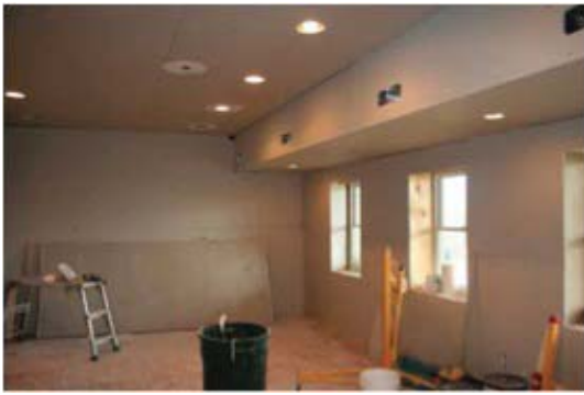
The room during the drywall stage, with a DriCore subfloor, a long soffit hiding the ductwork, and recessed in-ceiling can lights.
