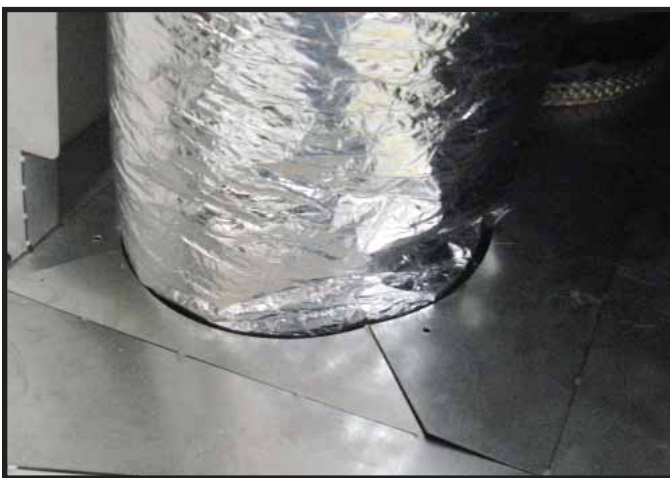
Figure 7.7. Bend Pre-cut Tabs Down.
