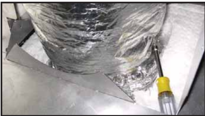
Figure 7.6. Install Insulated Flex.
