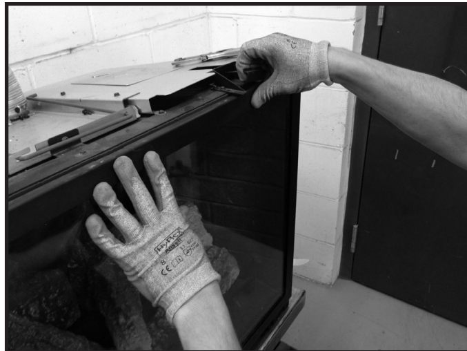
Figure 11.3 Release Glass Latches One at a Time
