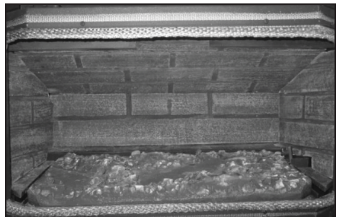
Figure 12.15 Finished Brick Installation
