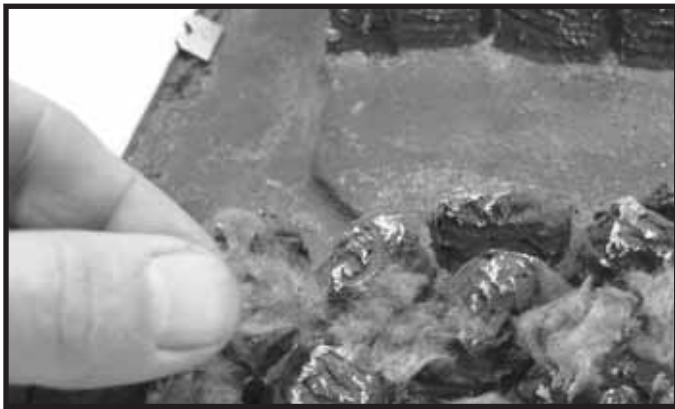
Figure 12.9 Placement of Embers
