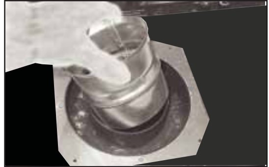
Figure 8.2 Remove the inner collar adapter.
