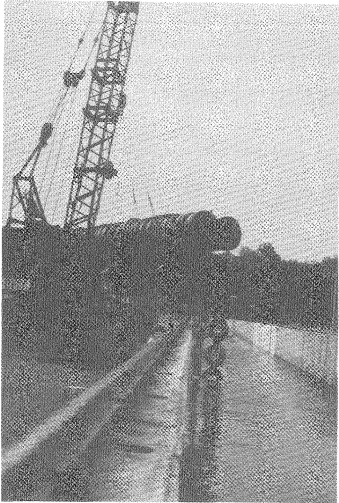
Fig. 19 Inserting PT-1 Breakwater
