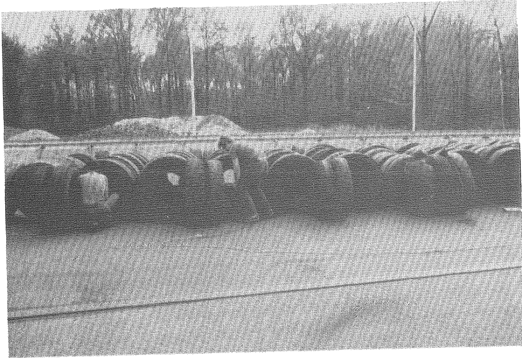
Fig. 10 Belts are Overlapped and Bolted Together
