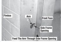
Figure 11 - Air Gate Arm in Front
