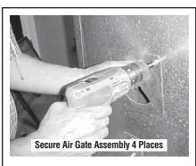
Figure 13 - Install Screws
