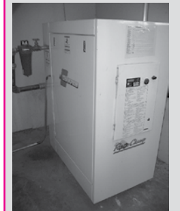
Champion Rotary Air Compressor w/Water Separator, Mdl. EFC99B, 25 HP, 125 PSIG, Mfg 11/03
