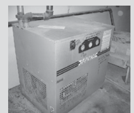
Arrow Pneumatics Inc Refrigerated Air Dryer, Mdl A-150-2, 10 HP
