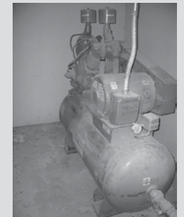
Champion Horizontal Tank Air Compressor, Mdl HRA25-12, Four Stage, 480 Volt, 200 @ PSIG, 650 F, 120 Gal Tank, 20 HP Motor
