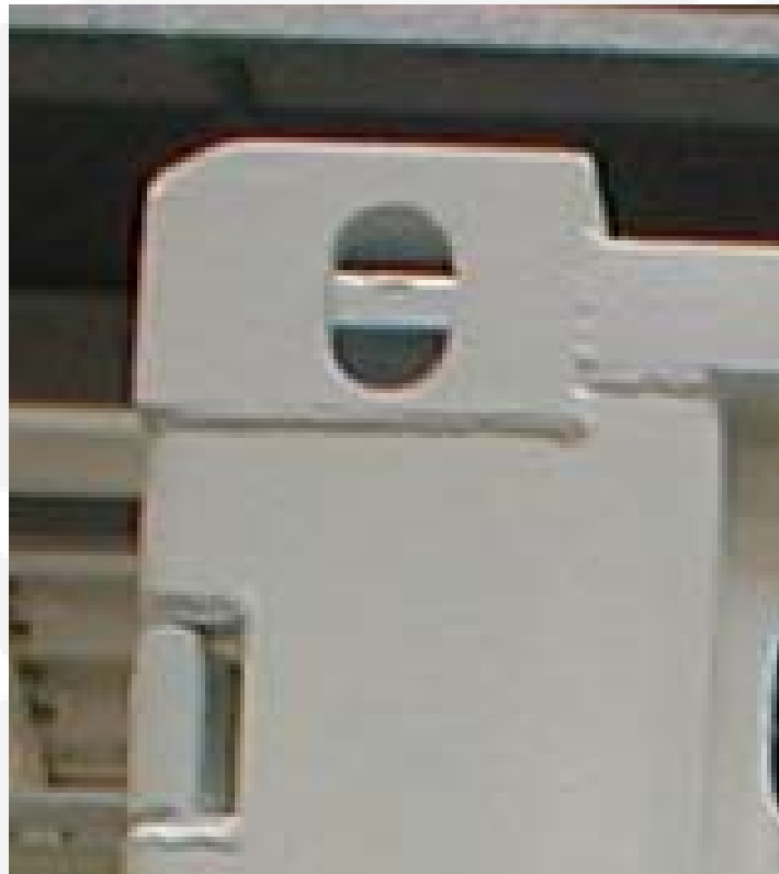
Figure 2-1 Lifting-eye (positioned at each top corner of the container)
