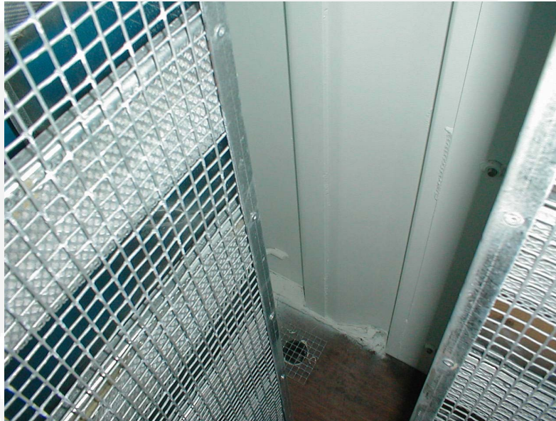
Figure 6-7 Drainage-hole position
