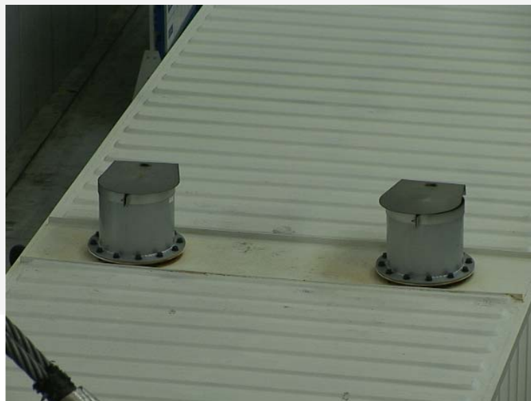
Figure 5-3 Exhaust Extensions
