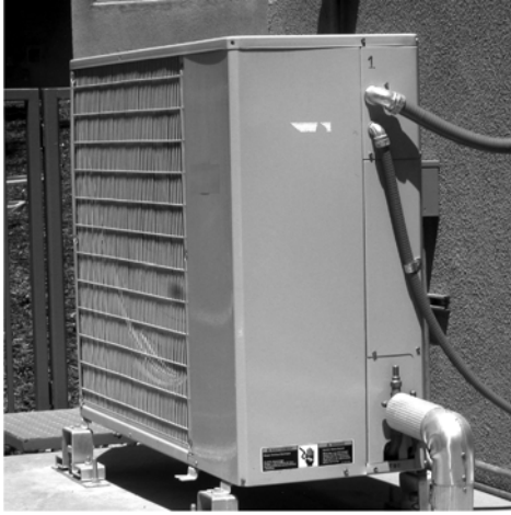
Figure 4-11 Outdoor condensing unit typically used with ductless split systems; it can also be used with ducted fan coil units.
