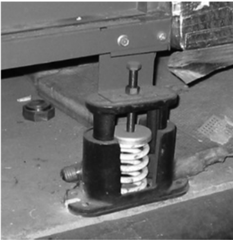
Figure 5-8 Cast-metal floor mount is prone to “short-circuiting” and should never be used. Instead, use a floor mount like that shown in Figure 5-6.
