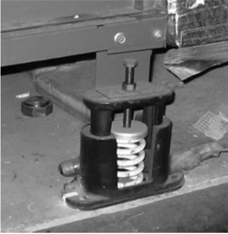
Figure 8-4 Restrained spring isolator with a “short circuit” between its baseplate and equipment mounting plate. This type of isolator has become obsolete and is not recommended for any type of HVAC equipment.
