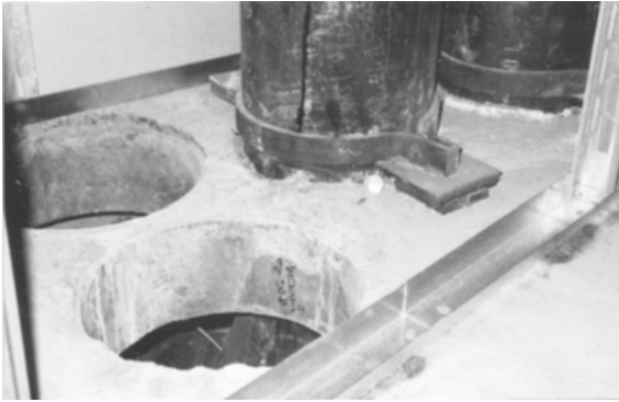
Figure 3-16 Vibration isolation for piping riser. The use of neoprene pads under the steel load-distributing plates indicates that the nearby occupancy was not very noise-sensitive. For more critical cases, steel spring isolators would be used.
