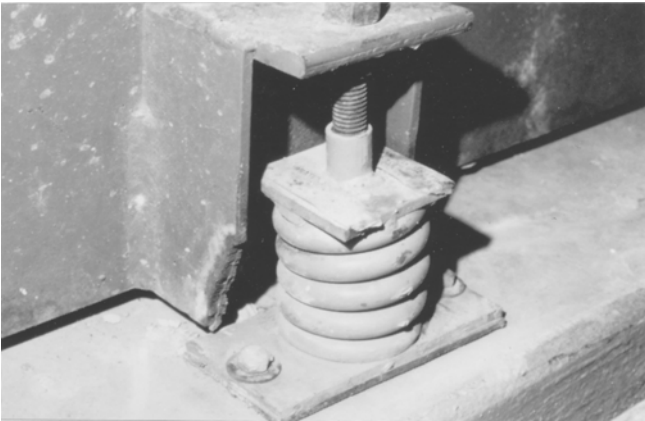
Figure 7-6 Overloaded free-standing floor mount. The overloading allowed the gussets welded to the side of the equipment frame to rest on top of the isolator baseplate. The lower right corner of the gusset was burned off to eliminate the gusset/baseplate contact. The proper action would have been to replace the overloaded spring with a stiffer one able to carry the heavy load.
