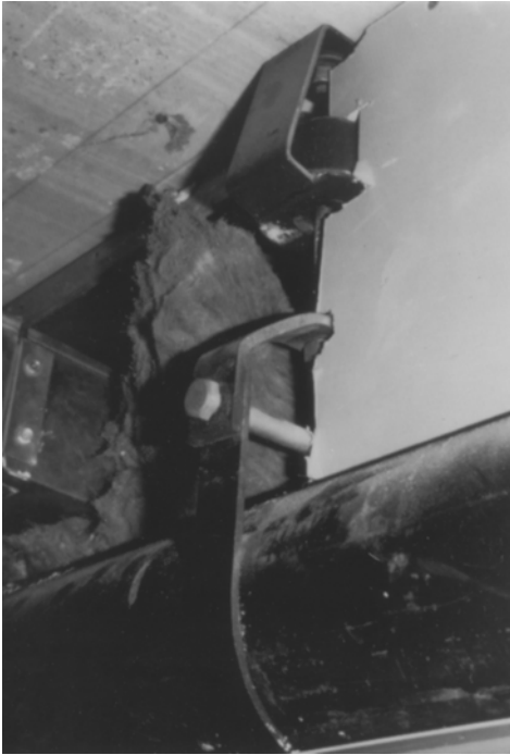
Figure 8-23 Improperly placed neoprene hanger. The drywall assembly forms a vibration transmission bridge across the isolator. This type of interference can be identified and corrected in pre-construction coordination meetings.
