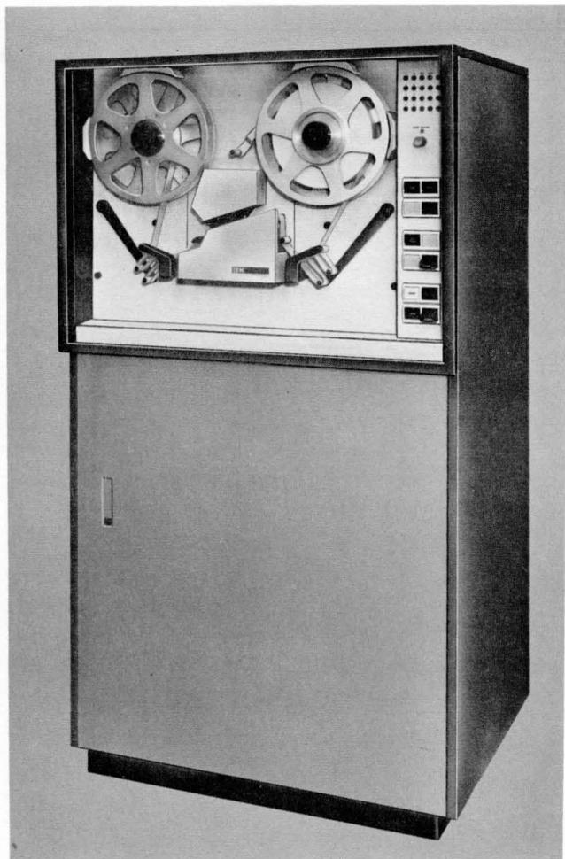
Figure E-25. IBM 1012 Tape Punch
