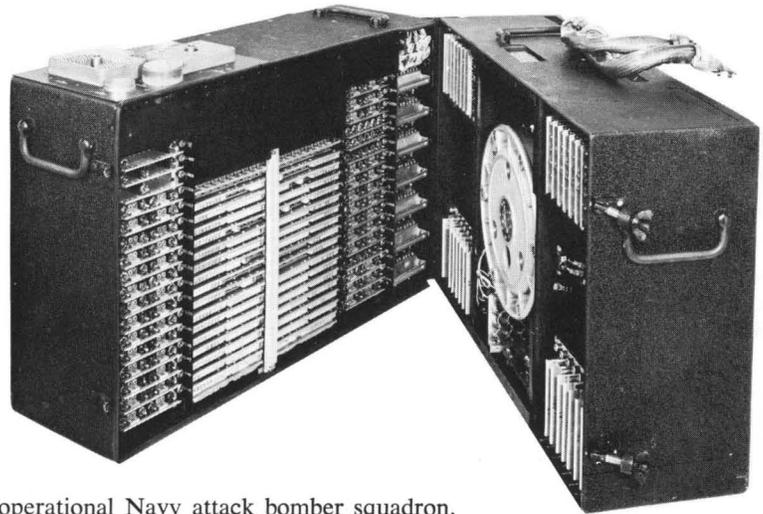
CP209 COMPUTER — first digital device performing bombing and navigation functions in an operational Navy attack bomber squadron.
