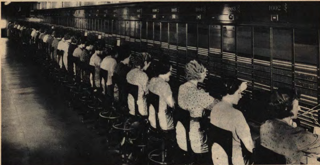
OUTWARD LONG DISTANCE SWITCHBOARD
