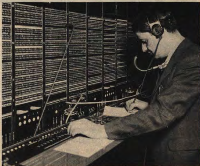
NO. 8 TEST AND CONTROL BOARD
