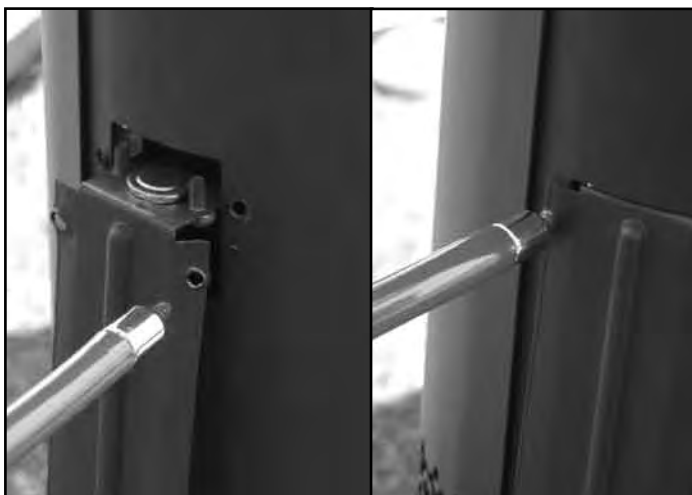
Figure 43: Spill switch installation.
