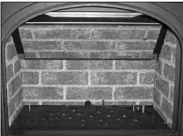
Figure 59: Side brick panels in place.
