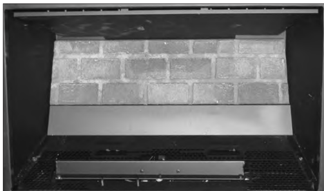
Figure 68: Back Brick Panel in Place.
