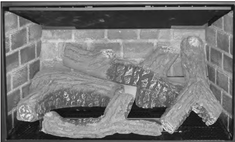
Figure 74. Fourth Stage Log Set Installation.
