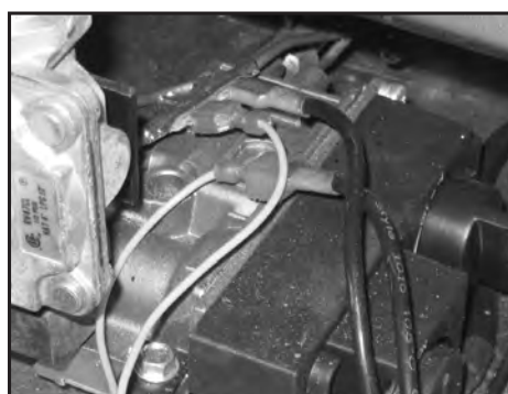
Figure 35: Spill Switch Wires Connect to Thermocouple.
