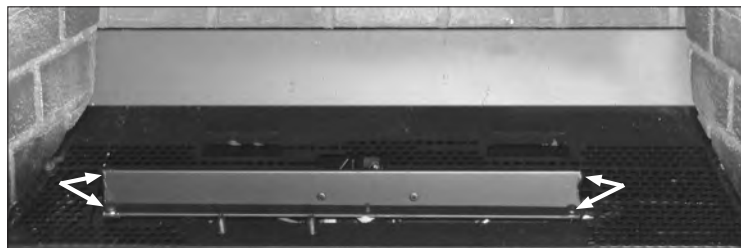
Figure 21: Unfastening Burner.
