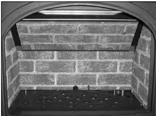
Figure 65: Side brick panels in place.
