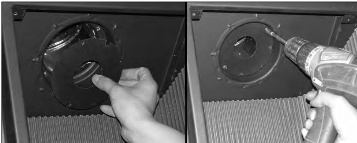
Figure 30: Flue Restrictor Installation.
