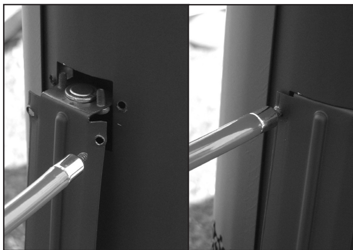
Figure 42: Spill switch installation.
