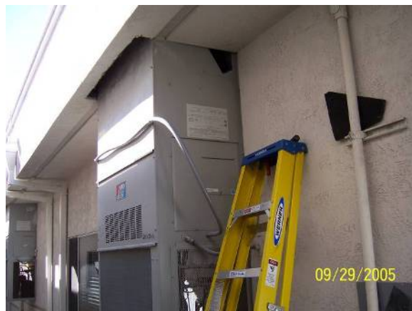
Figure 7. Example of a rooftop air conditioning unit in UVC study (top), schematic of a typical unit (middle), and example of a wall-mounted air conditioning unit in UVC study (bottom)
