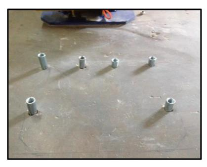
Drive anchor insert into hole with blunt hammer.
