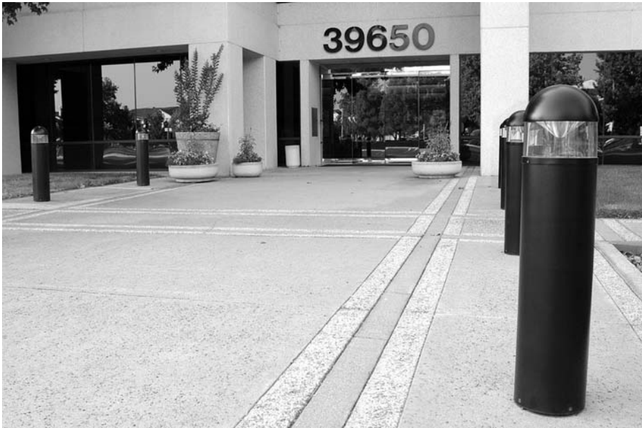
Figure 5-2 Sidewalks, lights, and landscaping can be used for protection.
