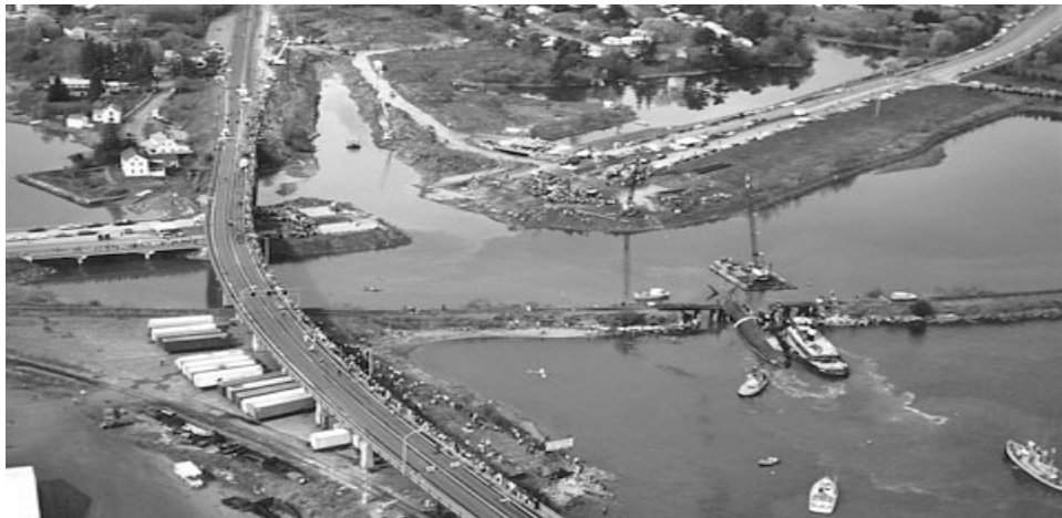
Entering rail cut en route to highway cut
