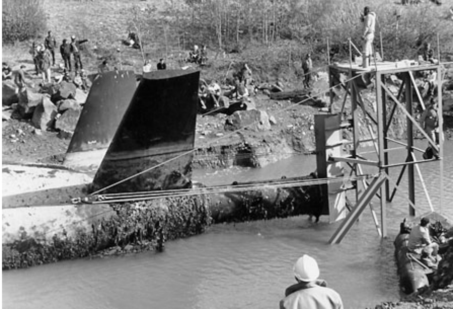
Positioned over the railway cradle
