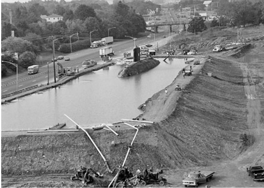
In position over the concrete cradle
