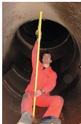
Repair in difficult conditions
