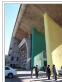
High Court front entrance
