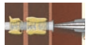
⑥ Starting from the back end, fill hole completely with mortar
