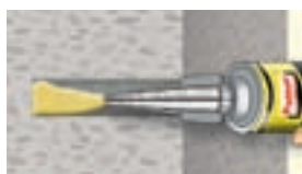
⑤ Starting from the back end, fill hole completely with mortar
