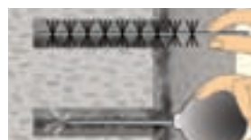
② Clean drill hole (blow out: 4x, brush out: 4x, blow out: 4x)
