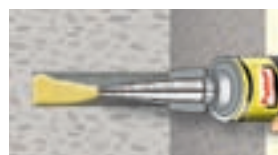
⑤ Starting from the back end, fill hole completely with mortar
