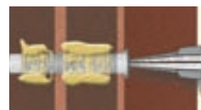
⑥ Starting from the back end, fill perforated sleeve with mortar
