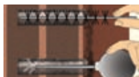
② Clean drill hole (blow out: 2x, brush out: 2x, blow out: 2x)
