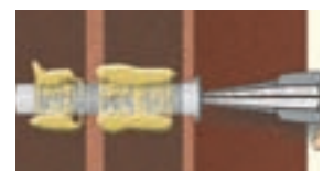
⑥ Starting from the back end, fill perforated sleeve with mortar
