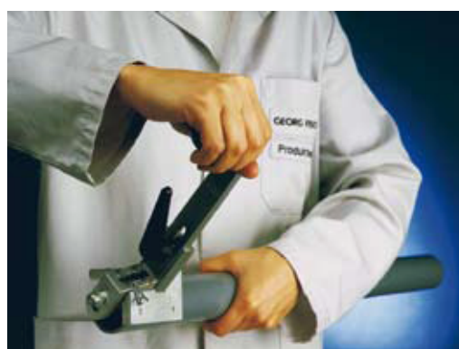
Chamfering the pipe
