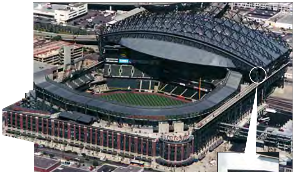
In less than 20 minutes, 96 Sumitomo Cyclo® Bevel Buddybox gearmotors help retract the 13,000-ton roof on Seattle's new Safeco Field.
