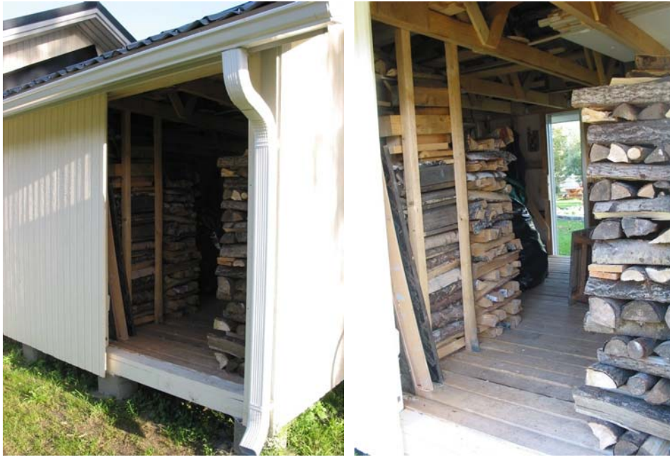
Figure 18. An ideal woodshed for storing one year's consumption of firewood. About 1.5-meter wide doorway allows firewood to be transported directly to the woodshed from the lorry. The minimum volume for Nordic conditions is 5 m 3 and in Southern Europe a few cubic metres. The floor has good ventilation when 50 x 100 mm sawn timber and 1 cm space between the floor planks are used. The front door is facing the building into which the logs will be carried. Photo: Lauri Sikanen.
