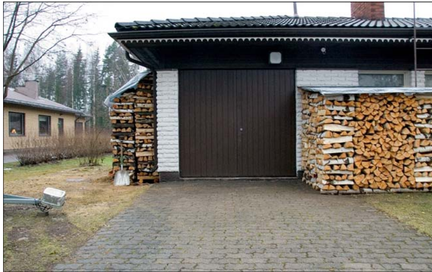
Figure 19. Firewood should not be stacked against the outer walls of buildings. Photo: Matti Alakangas.
