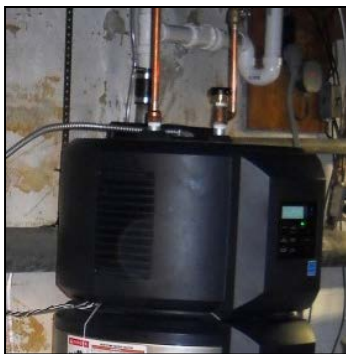
Figure 12. HPWH without heat traps
