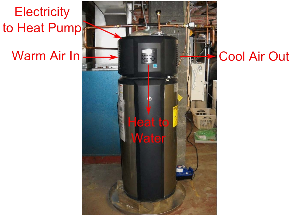
Figure 1. HPWH operation
