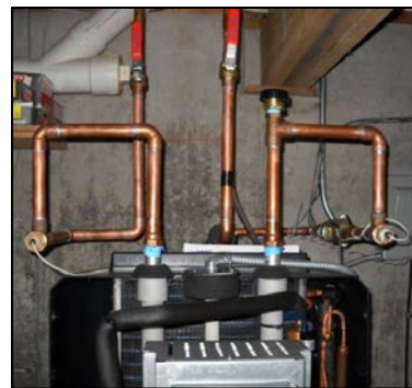
Figure 13. HPWH with heat traps
