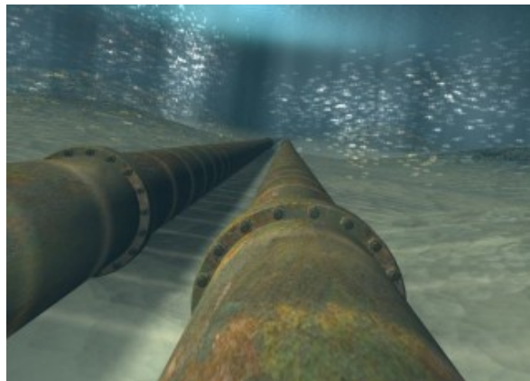
Corroded subsea pipeline ( http://subseaworldnews.com/2014/04/01/baosteel-yantai-delivers-subsea-steel-pipes-for-bohai-oilfield/ )
