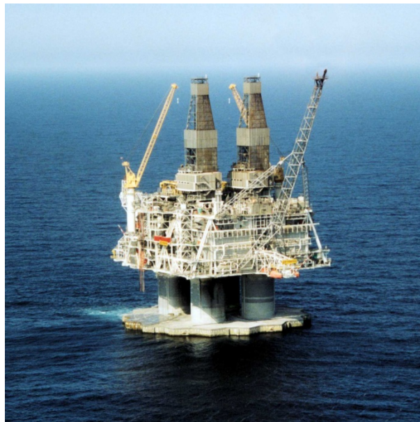
The Hibernia oil production platform, one of four installations located off the coast of Newfoundland ( www.hibernia.ca )
