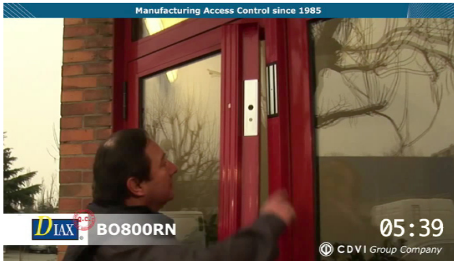
5 - Align the armature handle
