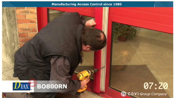
6 - Drill and fix the armature handle
