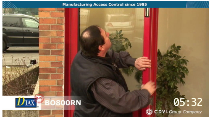
4 - Snap on the magnet housing cover
