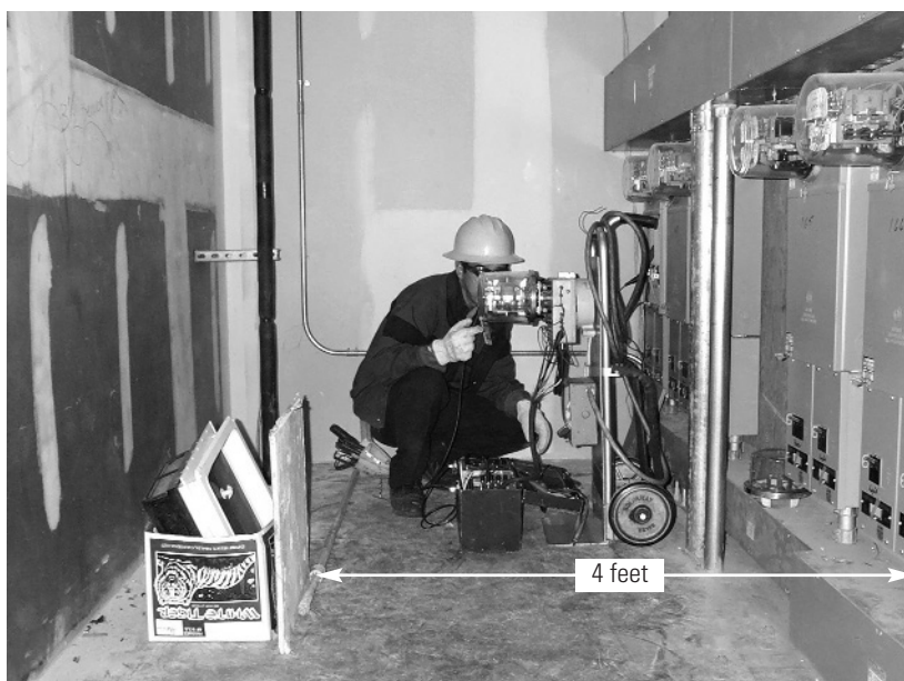
Figure 4-3. Meter electricians performing meter test. Notice the need for workspace clearance between the meter socket panel, and the pole on the floor.
