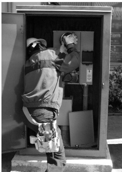
Figure 4-10. A free-standing meter enclosure must allow a 6-inch clearance at top and left side of meter socket to the enclosure rim, to allow the meter electrician to see and align the meter blades to the meter socket jaws.
