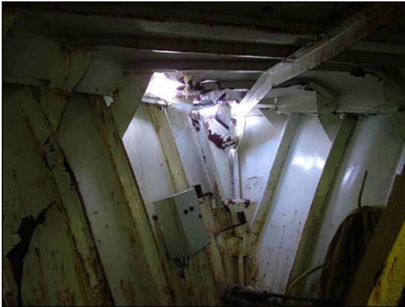
Damage to vessel
