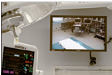
The 18-inch LCD monitor on the left displays vital statistics while the 40-inch LCD on the right is used for a number of functions including displaying dual images via the Extron MGP 462.
