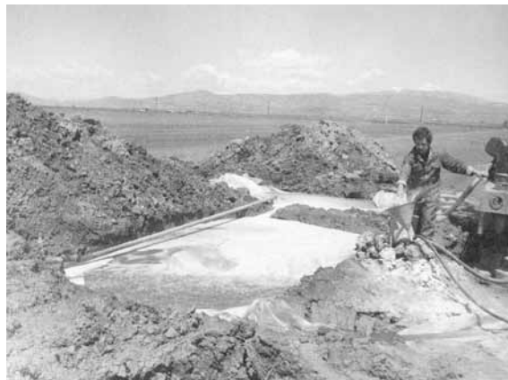
Example Photograph of a mud pit.
