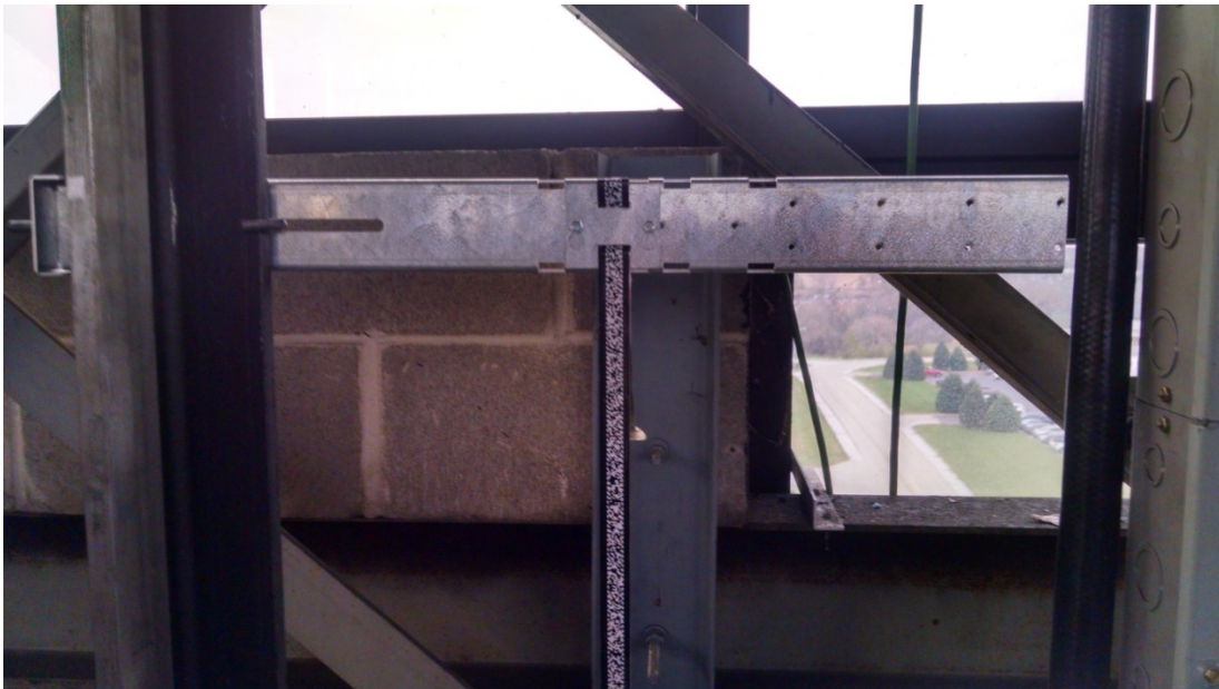
Figure 2.12: Encoded Tape Mounting
