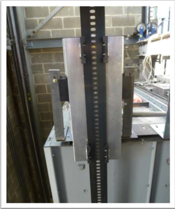
Figure 2.3: Typical Selector Installation
