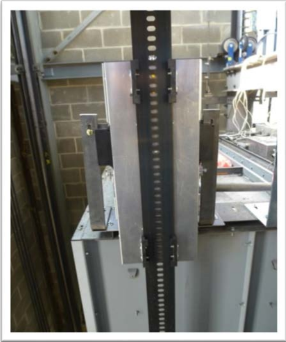
Figure 2.3: Typical Selector Installation
