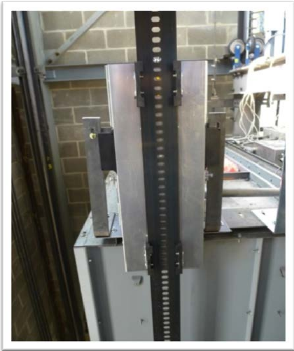
Figure 2.3: Typical Selector Installation
