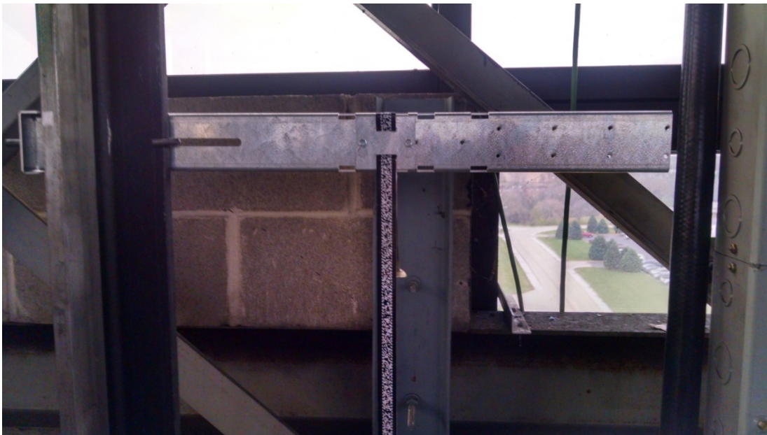
Figure 2.12: Encoded Tape Mounting
