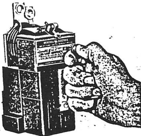
Fig. 15 Checking Travel Distance of Series Overcurrent Tripping Device
