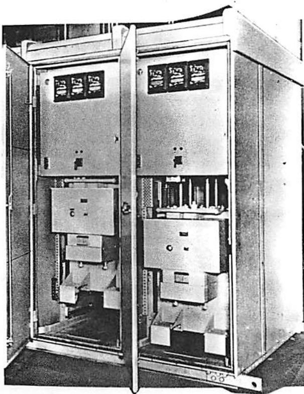
Fig. 2 Typical Outdoor Metal-clad Switchgear Equipment - Front View
