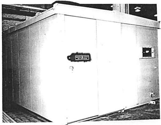
Fig. 3 Typical Outdoor Metal-clad Switchgear Equipment With Protected Aisle - Side View
