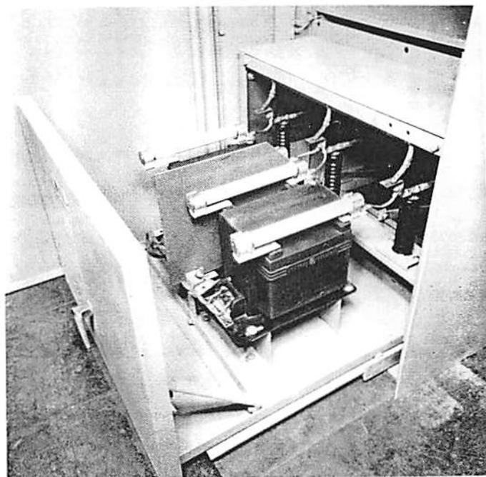
Fig. 12 Potential Transformer Rollout Shown in Withdrawn Position
