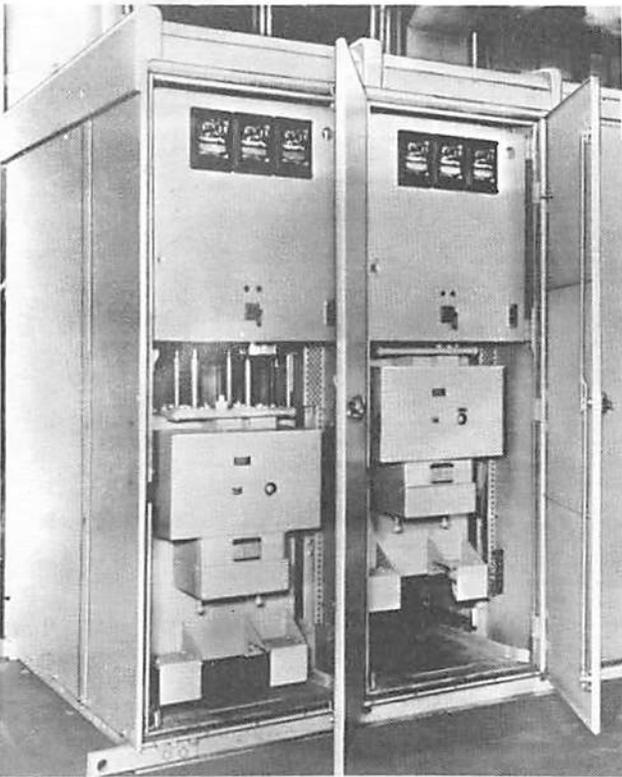
Fig. 2 Typical Outdoor Metal-clad Switchgear Equipment - Front View
