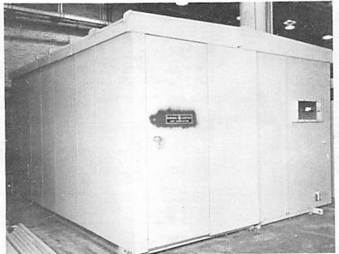
Fig. 3 Typical Outdoor Metal-clad Switchgear Equipment With Protected Aisle - Side View
