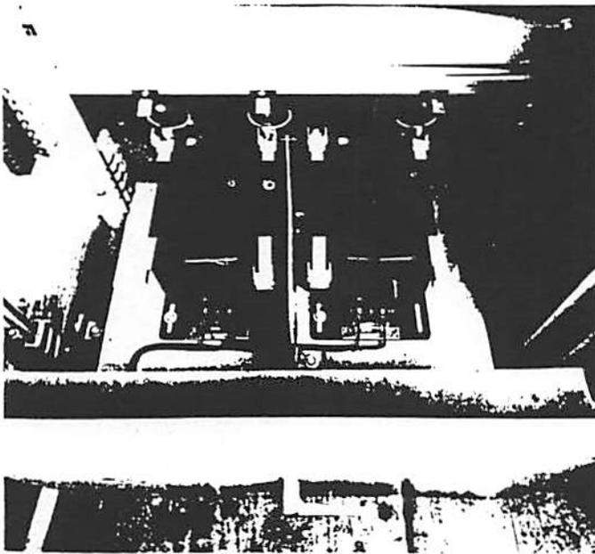
FIG. 12 POTENTIAL TRANSFORMER ROLLOUT SHOWN IN WITHDRAWN POSITION
