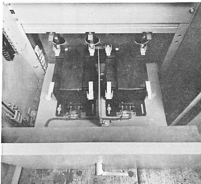
Fig. 12 Potential Transformer Rollout Shown in Withdrawn Position
