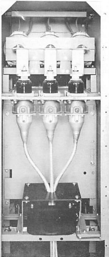
Fig. 42 Rear View of Unit Showing Through-Type Current Transformers
