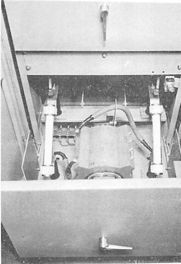
Fig. 16 Control Power Transformer Rollout Shown in Open Position
