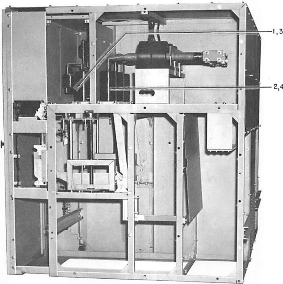
**Fig. 1 Metal-clad switchgear**
