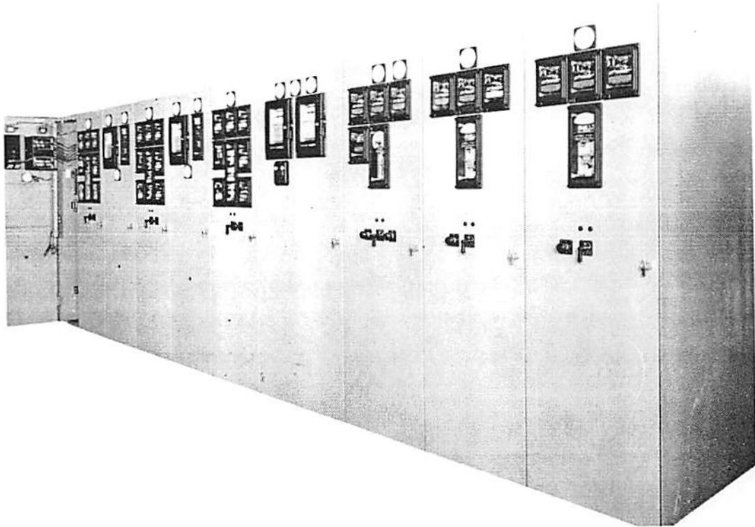
Fig. 1 Typical Indoor Metal-clad Switchgear Equipment
