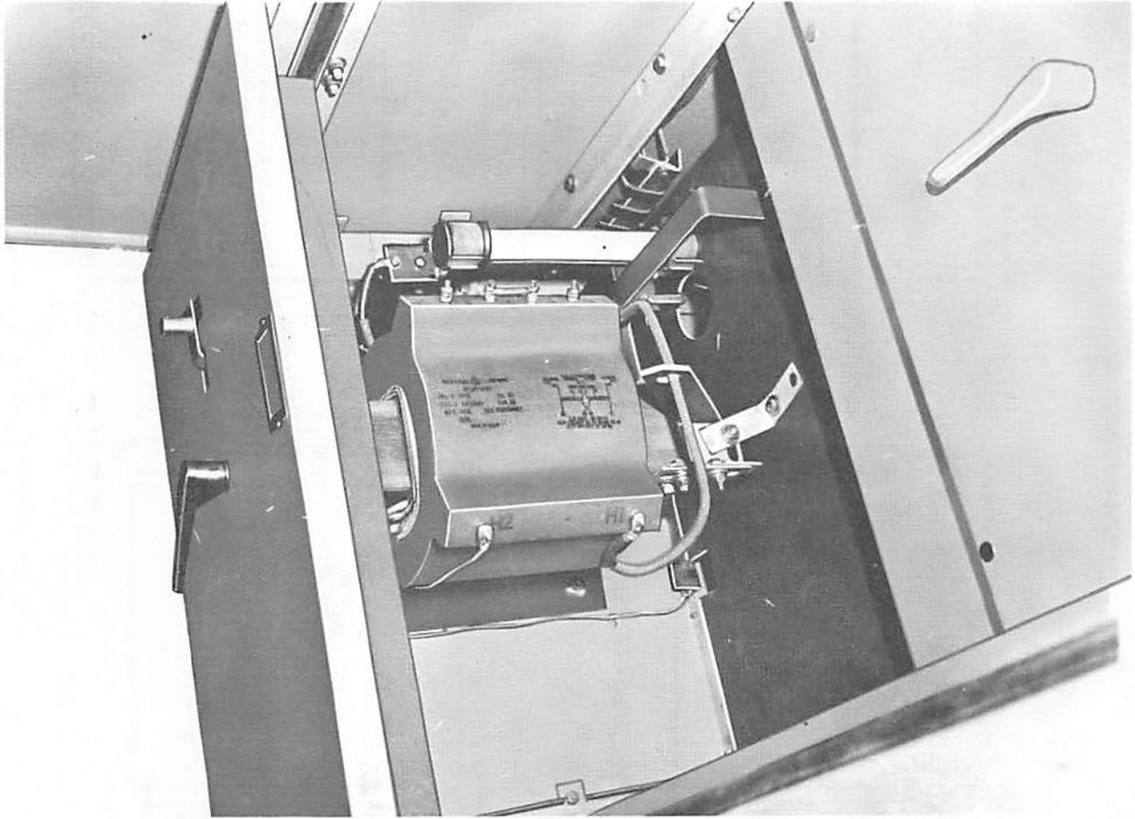
Fig. 16 Control Power Transformer Rollout Shown in Open Position
