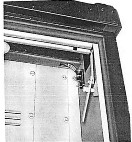
Fig. 17 Tandem Lock for Outdoor 13.8 Units
