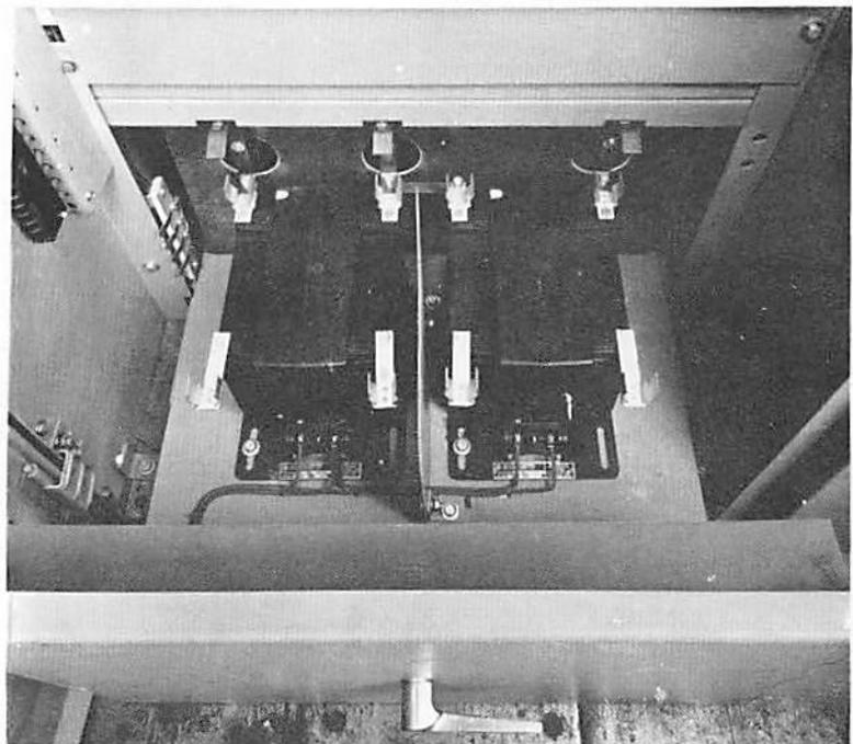
Fig. 12 Potential Transformer Rollout Shown in Withdrawn Position
