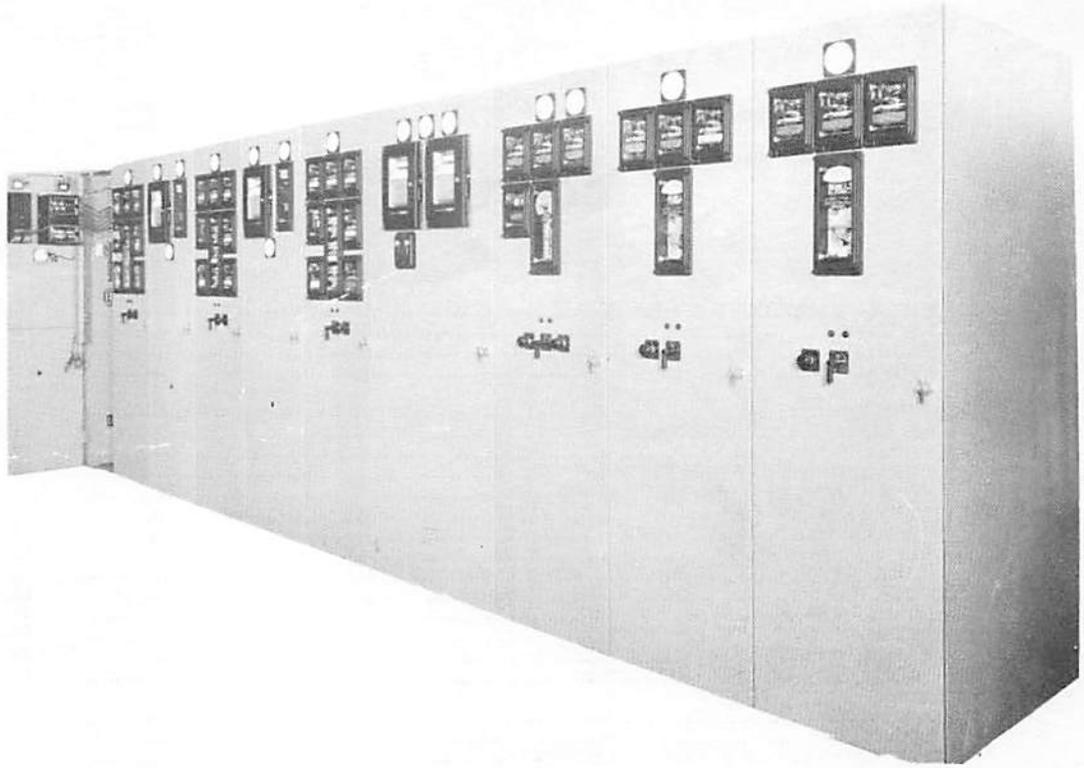
Fig. 1 Typical Indoor Metal-clad Switchgear Equipment
