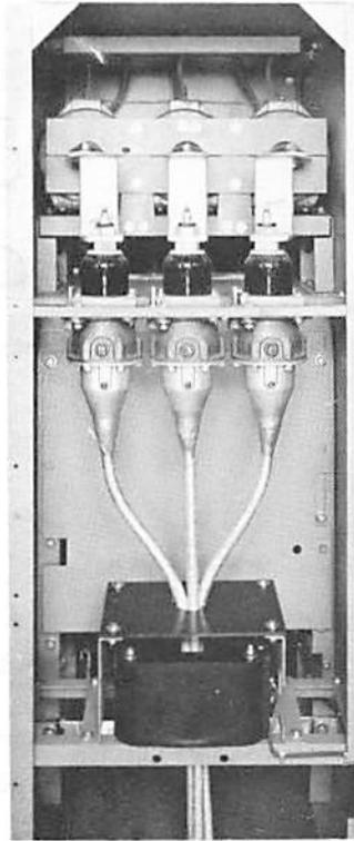
Fig. 27 (8026383) Rear View of Unit Showing Through-Type Current Transformers
